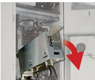
Modules can be popped out towards the front
