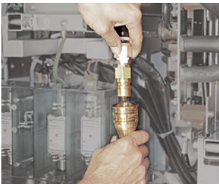
Liquid cooling can be disconnected quickly and without any spilling using quick-release couplings
